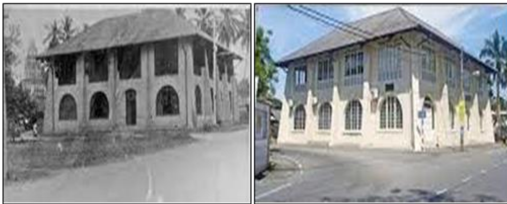
Figure 4: Bank Kerapu in Kota Bharu, Kelantan was converted to War Museum Sources: muzium.kelantan.gov.my
