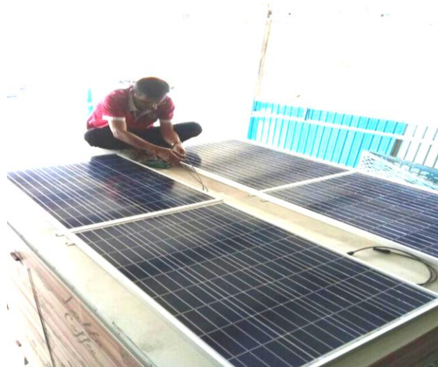
Figure 2: Installation of solar panels
